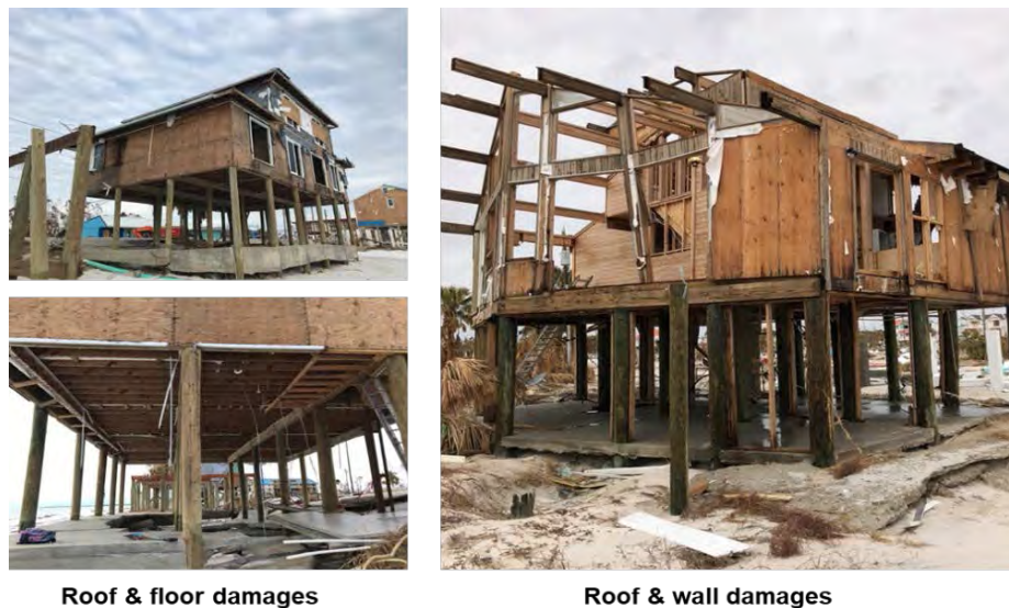
Figure I-1 Single-story houses elevated by 8 ft and 9 ft (wall, roof and floor damages) Hurricane Michael (2018) Mexico beach, Florida (Alipour et al., 2018).
