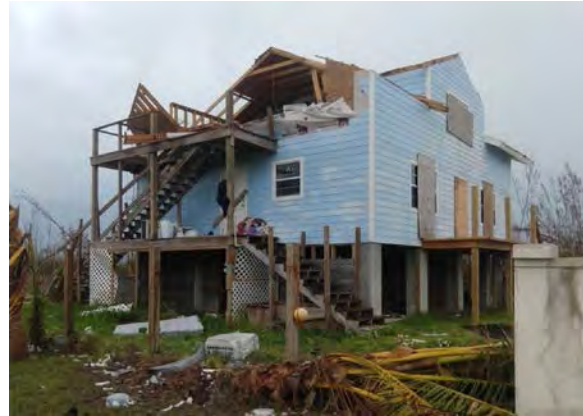
Figure I-2 Two-story elevated house after hurricane Dorian.
