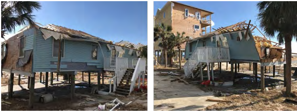
Figure I-4 Coastal house elevated by 7 ft with aspect ratio > 2 severely damaged Hurricane Michael (2018) in Florida
