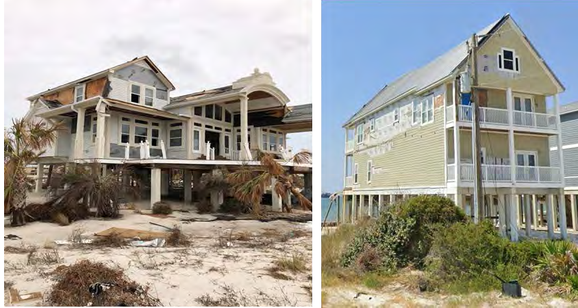
Figure I-3 Two-story houses elevated by 8 ft (wall, roof and stairs damages) Hurricane Michael (2018) Mexico beach, Florida (Alipour et al., 2018)
